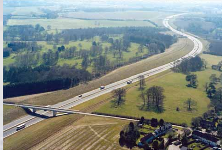
A10 Wadesmill Bypass: Fitzpatrick's value engineered design meant that arisings were almost totally absorbed into the embankments and landscaping. This significantly reduced cost and disruption.
