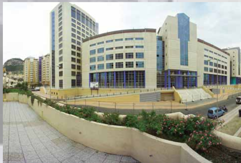
Gibraltar General Hospital: This Fitzpatrick/Rotary International JV is one of Gibralta's largest construction contracts providing operating theatres, wards, intensive care units, accident and emergency room, hydrotherapy centre, maternity, day-care and paediatric centres, and medical training facilities.
