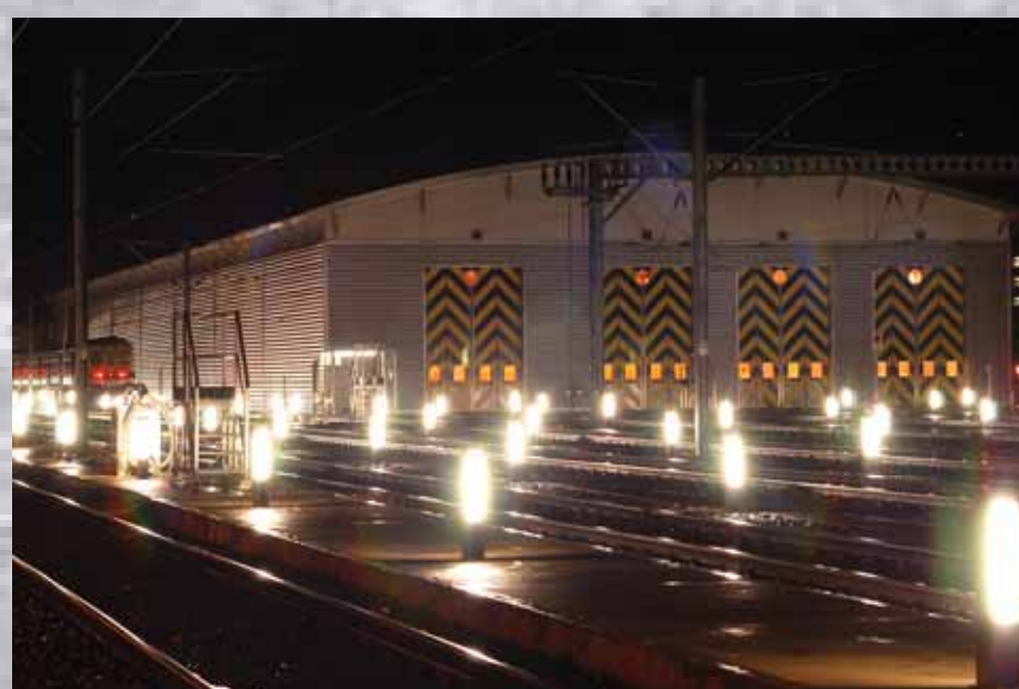
Bedford Light Maintenance Depot: Awarded 'Achievement through Team Work' at the Railway Industry Innovation Awards. Fitzpatrick has recently been awarded the £87m Ashford/Ramsgate LMD.
